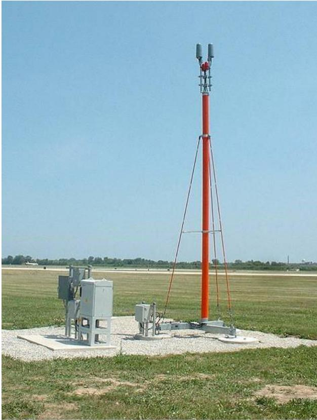
**Figure 2 MSS Sensor (Remote Unit)**
