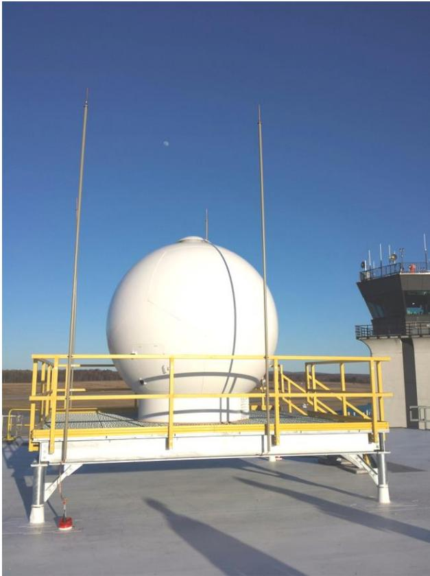
**Figure 3 LSTAR Radar Installed at Griffiss**
